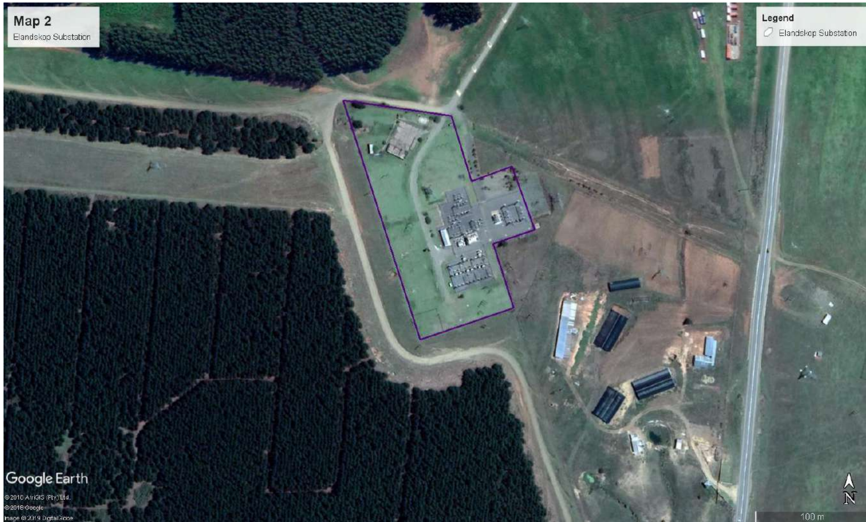
Figure 2: Elandskop Substation (Purple), (Google Earth Imagery, 2018)
