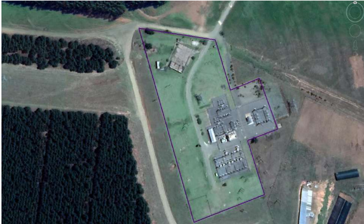
Figure 7: Aerial Snapshot of the Existing Elands kop 88kV Distribution Substation (Google Earth Image, 2018)
